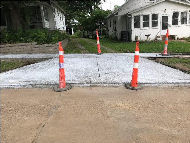
New driveway apron on West side of Burgess Ave.
