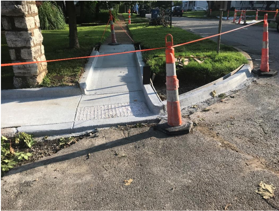
Northwest corner of Oakland and Marion Ct.
