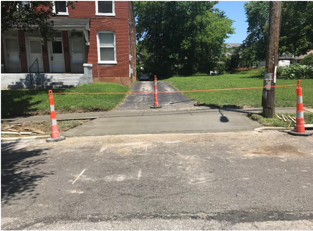
New driveway apron on Lohmeyer Ave.
