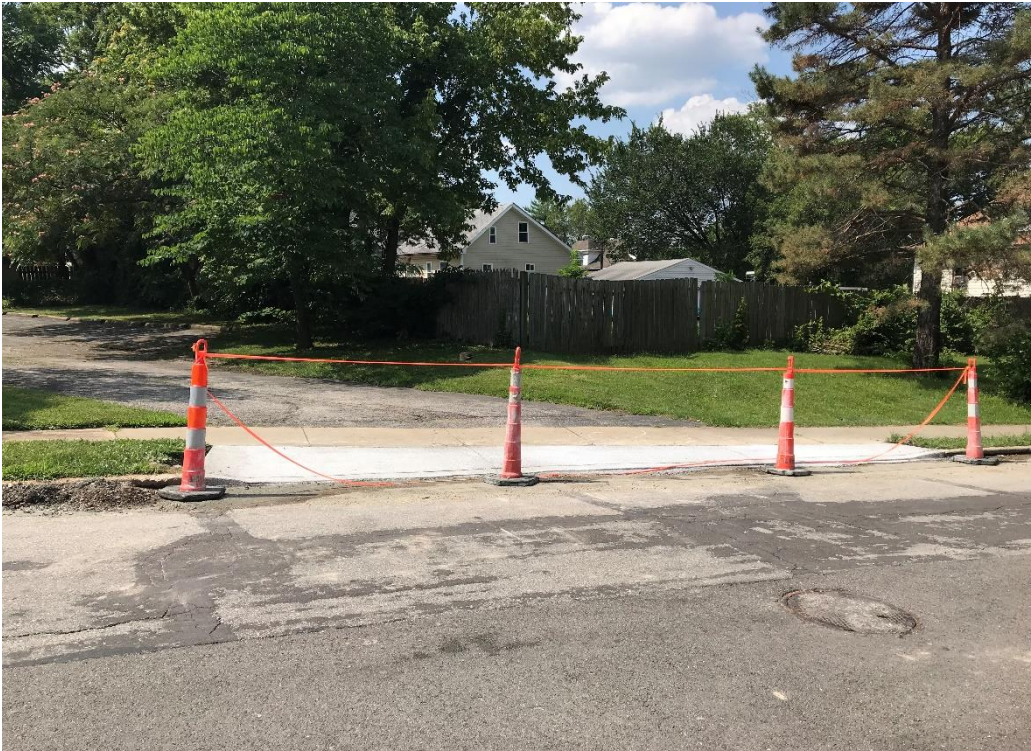
New driveway apron on Lohmeyer Ave.
