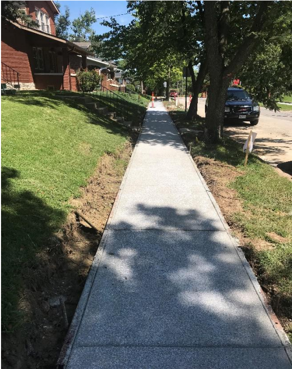
New sidewalk on Richmond Place between Oakview Terr. and Sutton Blvd.
