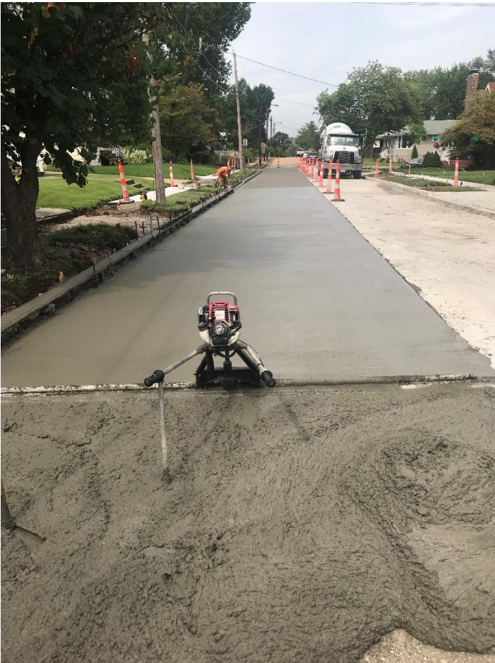
Start of concrete pour on Friday. Richmond Ave. facing west.
