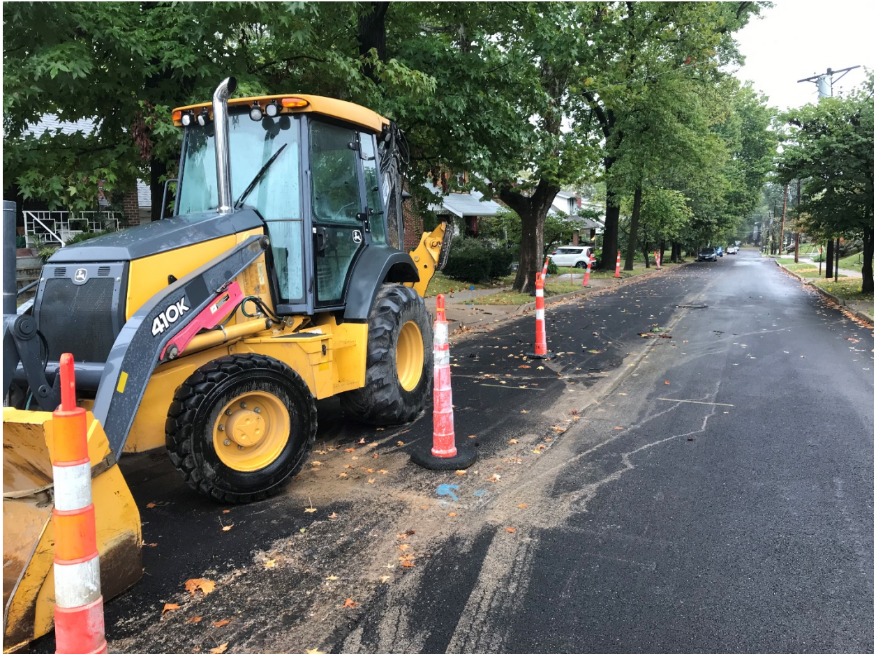
The street is saw cut and ready to be excavated.
