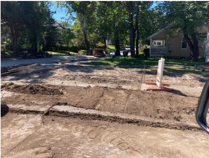
Cleaned up corner at Kensington and Commonwealth
